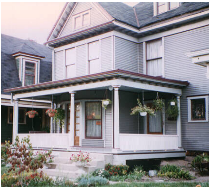
The same house 4 years later. Since this picture was taken, a new roof has been installed as well.
